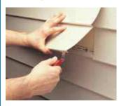
Wedge tip under the bottom end of overlapping panel and hook on the back lip of buttlock in one easy motion.
